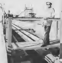
Night Shift Coordinator Adrien stands over pipe banks. Night Shift Coordinator Adrien stands over pipe banks.
